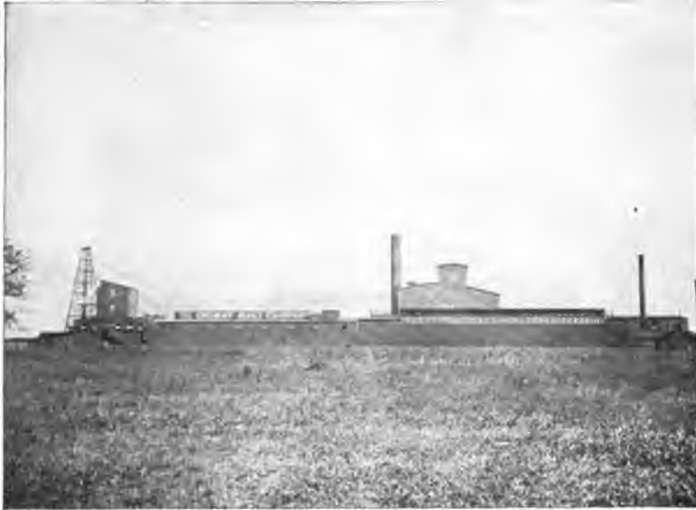
A. PLANT OF THE DELRAY SALT COMPANY, DELRAY, MICHIGAN.
